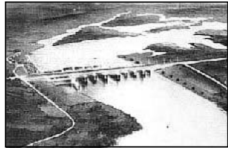
The Pak Mun Dam
